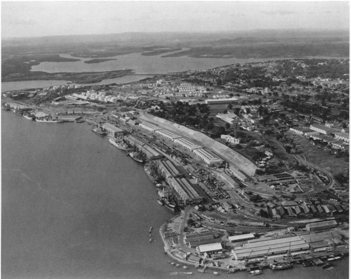
Fig. 10: A detailed view of the Kilindini deepwater wharf area on the western side of Mombasa Island. Lower right section shows a part of the lighterage wharf. In the distance can be seen the Makupa causeway and the expanse of Port Tudor.
