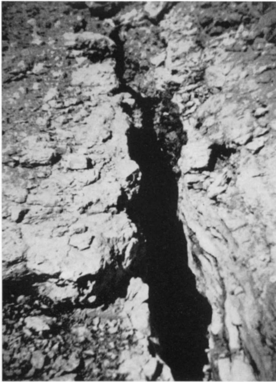
Photo 1: Narrow and lengthened cavities. Note in upper part a diaclases with direction N 70° W — S 70° E.
