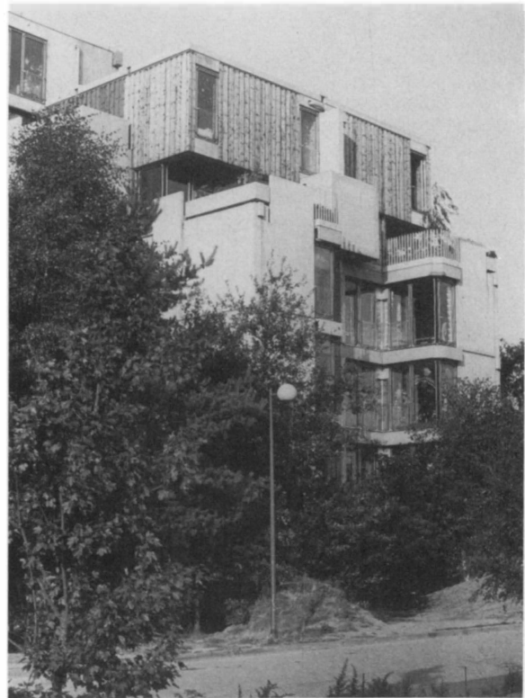
Photo 5: Habiflex. Note the removable nature of the glass panels around the enclosed balconies. (Source: H. KREHL and Partner)
