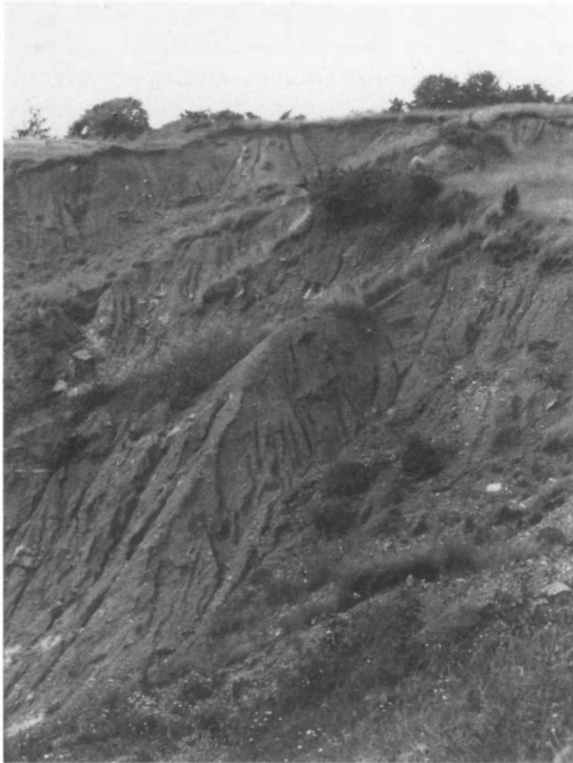
Photo 1: Part of the headscarp (in the background) and of the lateral scarps of a "rotational earth slump" on the southern slope of the valley. The process of landsliding is still actual, with regressive headward and lateral enlargement of the scarps. Linear erosion on the slump scarps intensifies the erosive slope destruction
