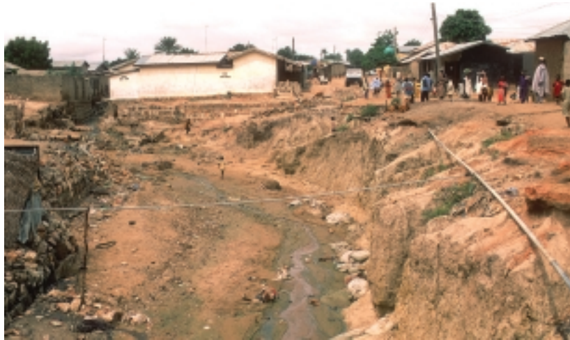
Photo 1: The old town of Gombe: isolation of wards by gully erosion and destruction of infrastructure Source: BALZEREK 2000
