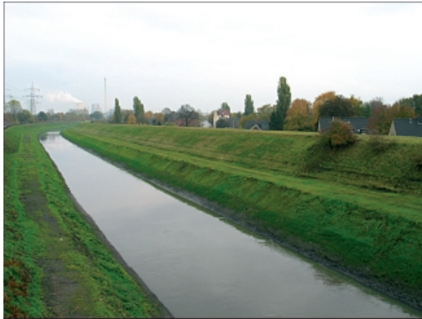
Photo 1: River Emscher in Herne (Photo J. HERGET). Due to land subsidence caused by coal mining no wastewater removal network by underground pipelines could be established in historic times. In the beginning of the 20 th century it was decided to modify the entire River Emscher catchment to an open wastewater removal system. Hence, the channel was straightened and dykes were built at the shorelines to protect the densely settled area of subsidence from floods.
