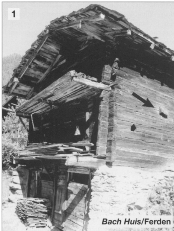
Photos 1, 2: Comparison of the Bach Huis (AD 1502, tree-ring dated) with a ridge-transverse main room beam (black arrow) and the Jeiziner Huis (AD 1591, by inscription) with ridge-parallel beams (white arrow). These construction techniques are representative for differing construction periods
