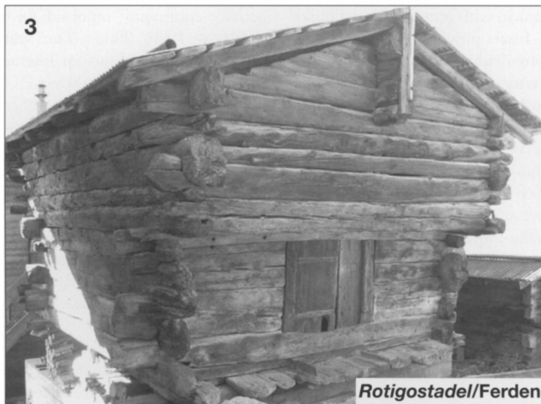
Photo 3: The oldest, originally preserved shed within the Lötschental ( Rotigostadel in Ferden, AD 1302)
