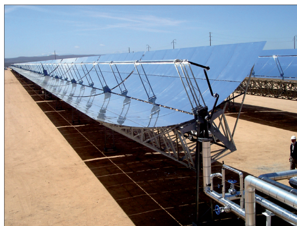
Photo 2: CSP parabolic-through technology. Source: Solar Millennium
