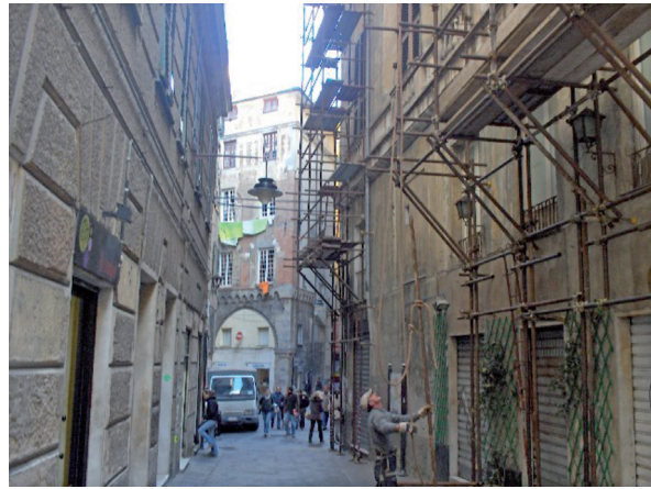
Photo 3: Restauration of the historical centre
