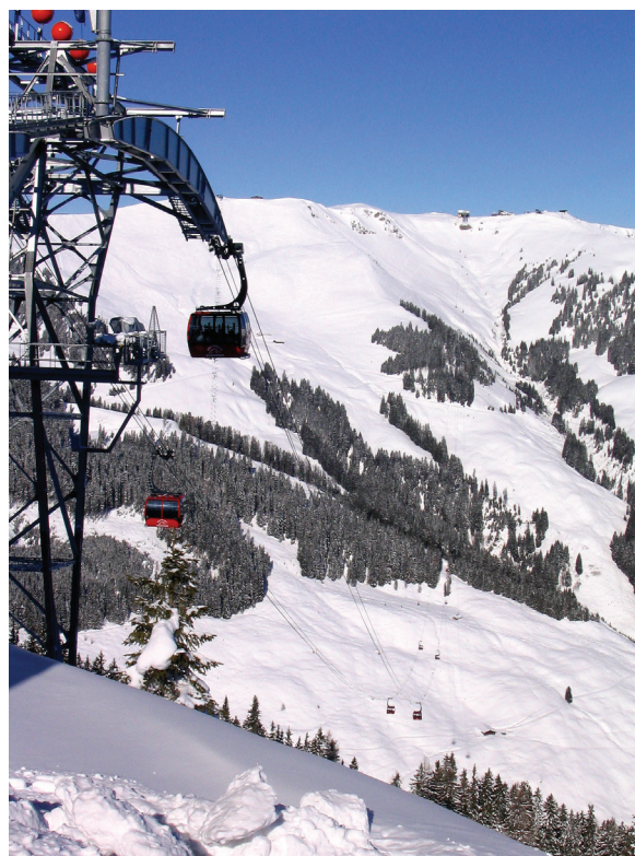
Photo 1: Since the season 2004/05 the Tricable Gondola Detachable „3-S“ (Kitzbühel, Tyrol, Austria) links the two formerly separate ski areas Hahnenkamm-Pengelstein and Jochberg-Pass Thurn and doubles the accessible ski area. The glass bottom-gondola #1 unveils a daunting view of the ground a steep 400 meters below. Photo by Michael Neufeld 2005
