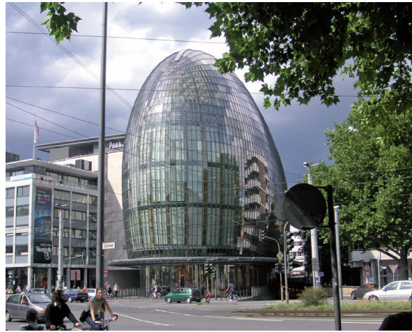
Photo 2: Retail building projects: "Peek und Cloppenburg" in Cologne (Photo: C.-C. Wiegandt)
