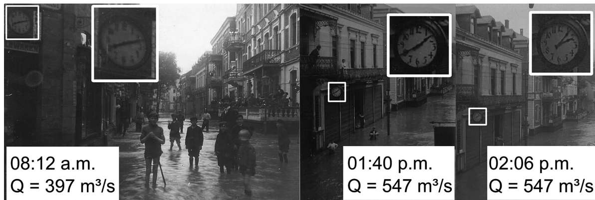
Fig. 7: Photographs documenting the water level of the flood event of 1910 in Neuenahr during June 13 th
