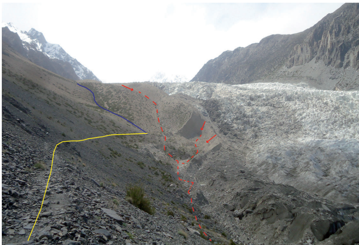
Photo 3: Currently working (blue) and desiccated (red arrows) water diversion channels sourced by Passu Glacier. The recent water intake is more than 5 km upwards from the settlements and has to pass through landslide-prone sections. Therefore, underground pipelines have been used (yellow line) to protect the channel against mass movements. (Photo: SITARA PARVEEN 2013)
