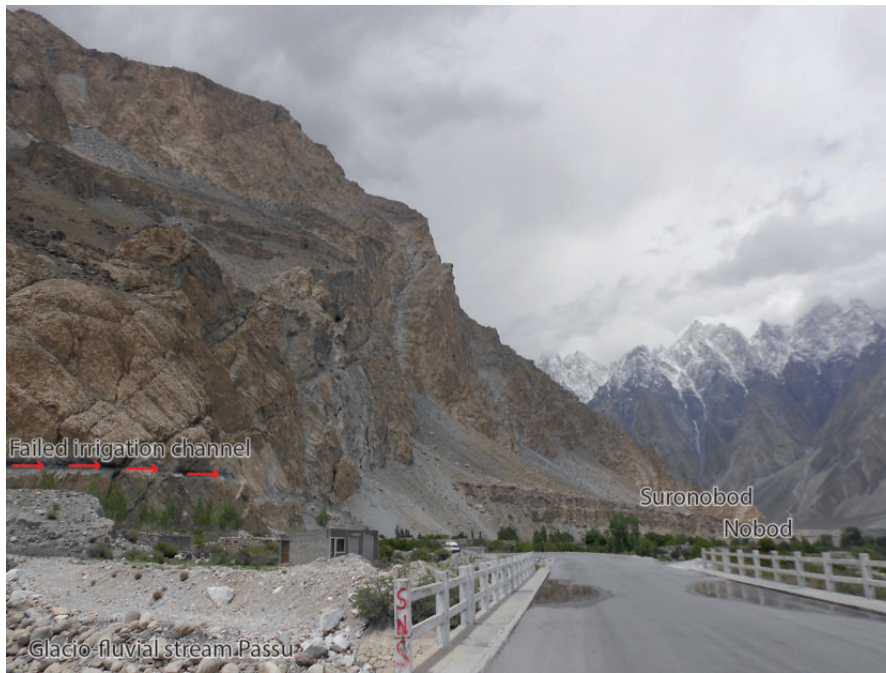
Photo 1: Failed irrigation channels to divert water from Passu Glacier to Suronobod Passu. (Photo: SITARA PARVEEN 2013)
