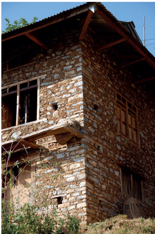
Photo 2: Low-Strength-Masonry (stone in mud unfinished without plaster) (Photo: J. ANHORN 2012)
