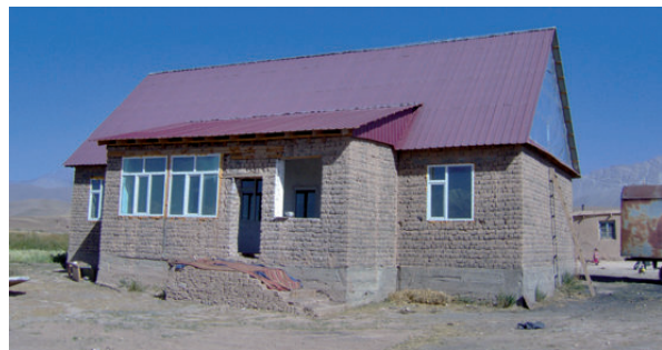
Photo 6: House under construction (117 m 2 living area) (Photo: C. SONNTAG, 11 September 2012)
