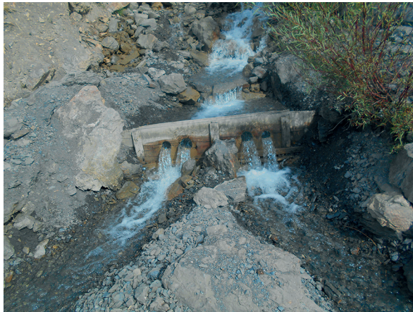
Photo 1: Main Nerwal of Kushum - an unmodified indigenous water allocation device
